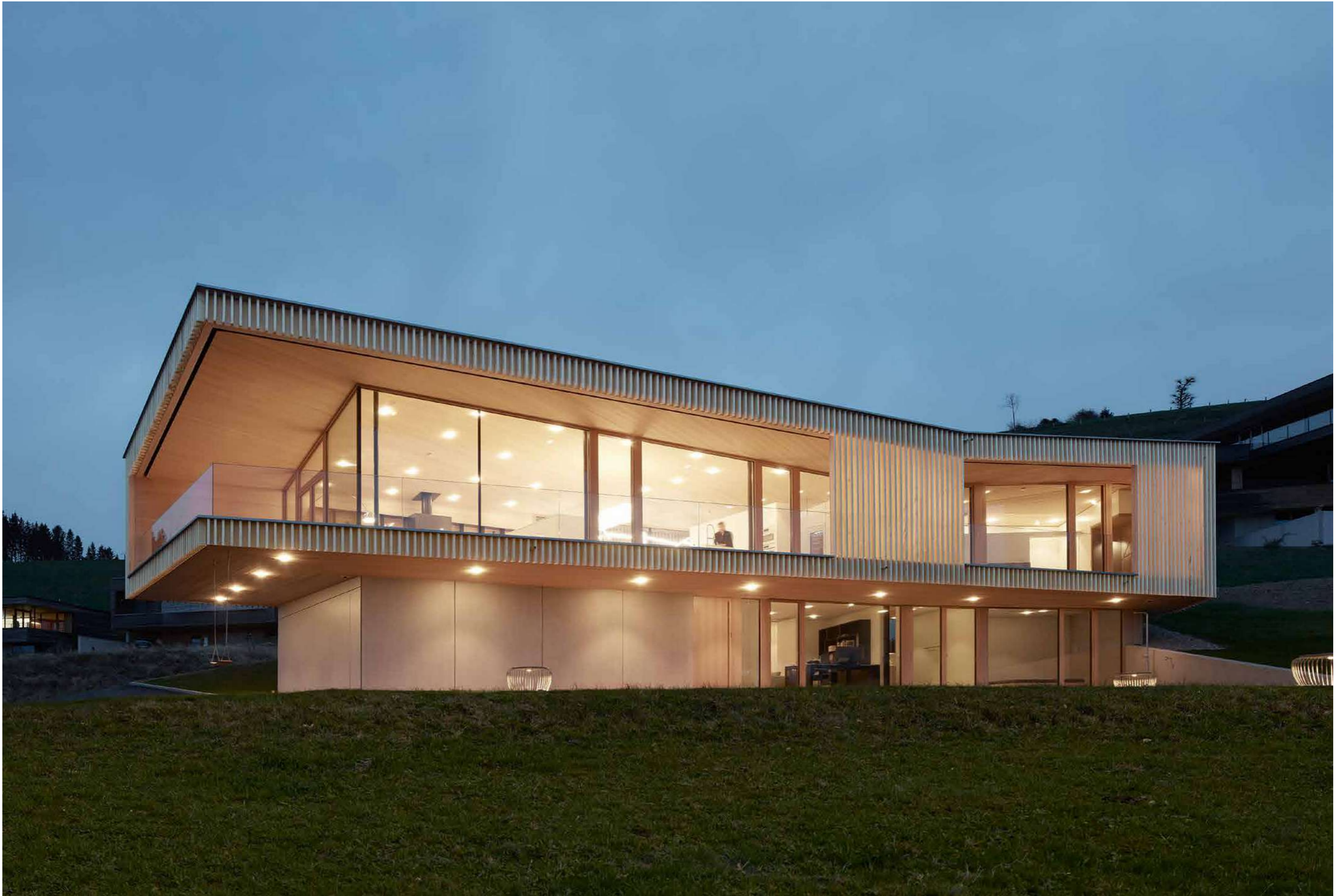
House on the Eichenberg (AT) Nimbus luminaires inside and outside: discreet appearance and consistent design
